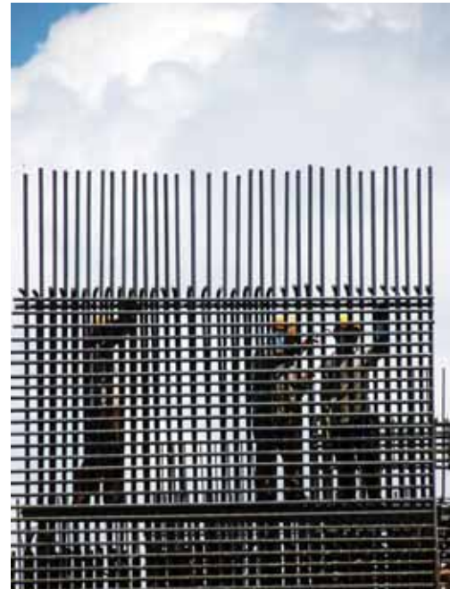
Steel Reinforcement Bars – Application on construction site
