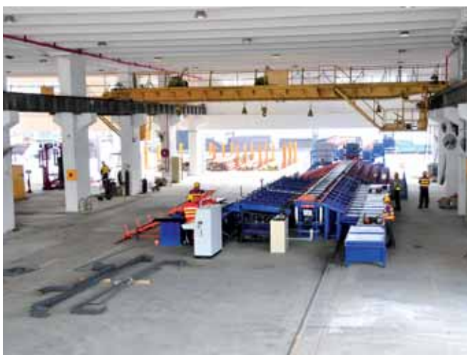
Steel Rebar Processing Centre in Tai Po, Hong Kong
