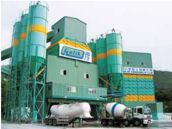
Ready Mixed Concrete Plant in Siu Ho Wan, Lantau Island, Hong Kong
